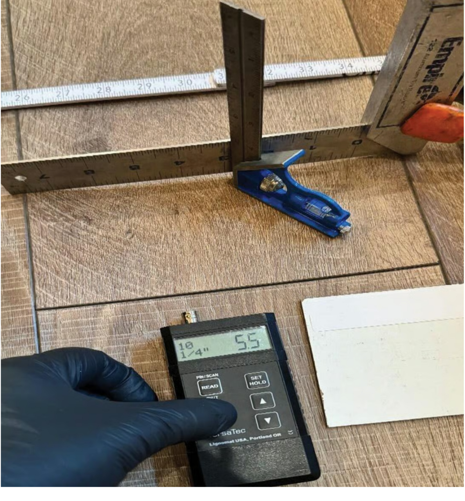
For example, in one inspection, edge curling was visibly confirmed using a ruler placed across the planks. Moisture readings at that spot with a Ligno-VersaTec from Lignomat showed a value of 5.5. Photo: Lignomat.
