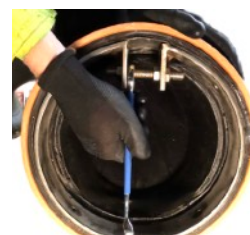
Tightening the clamp compresses the rubber to the pipe
