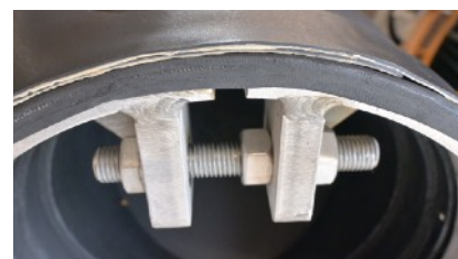
Check the valve O.D. snugly fits within the pipe I.D.
